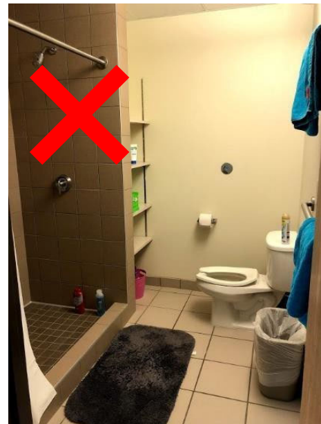
This is not ready .
